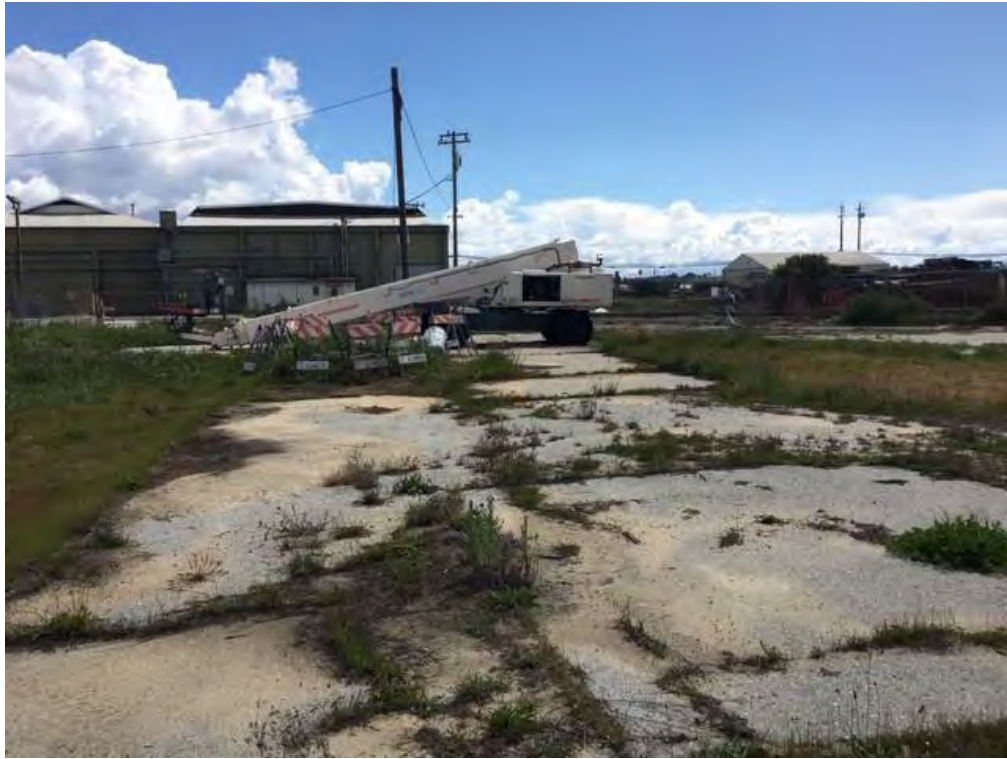
Figure 7. Degraded Asphalt in the Project Site
